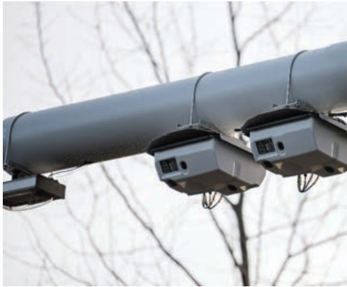
Image 3: Example of the redundant VDX sensor positioning at the portals
