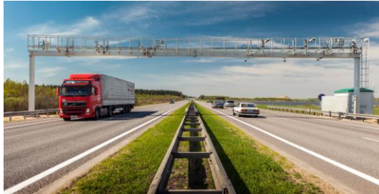
Multi-Lane Free-Flow Tolling
