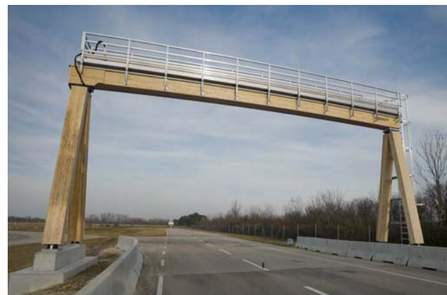
The Green Gantry by Kapsch, made from timber
